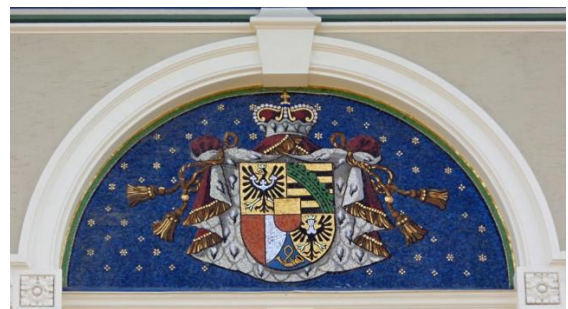
The national emblem of Liechtenstein on the building of the original seat of the Provincial Assembly in Vaduz (now government).
